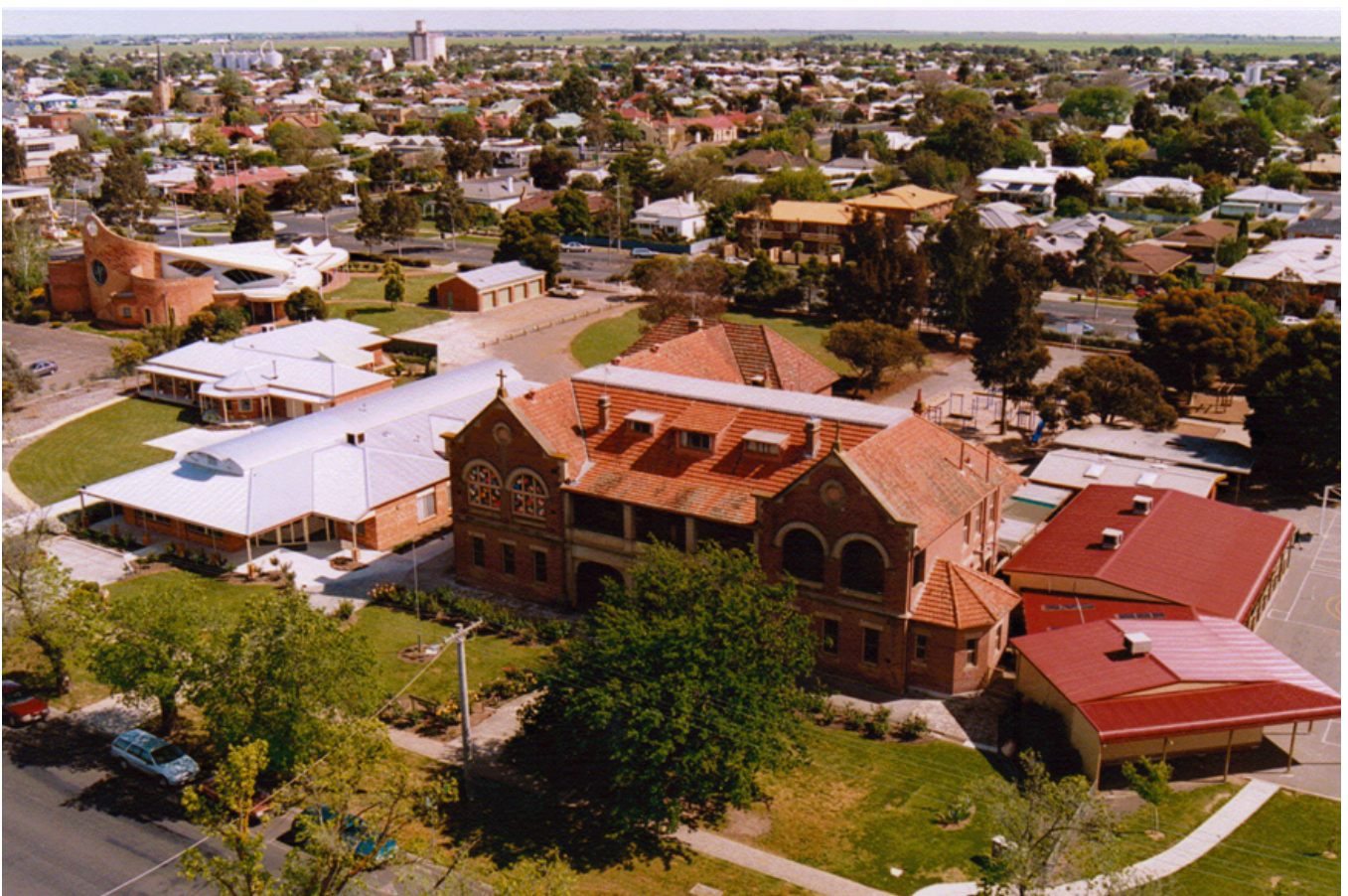
Former Brigidine Convent and Ss Michael and John's Primary School Buildings
